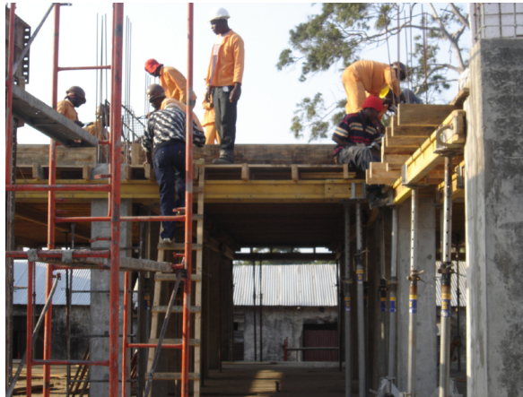
Figure 1.2.1: A building being constructed
